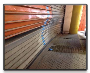
A damaged bottom bar and bottom slats are usually the result of repeated impacts to the door. The door can be further damaged by continuing to use it when there is slight damage, but not enough to inhibit operation. Typically, the door will continue to take the repeated force until at some point it will no longer operate.
